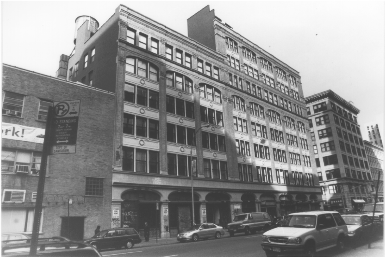
Lafayette Street Facade
