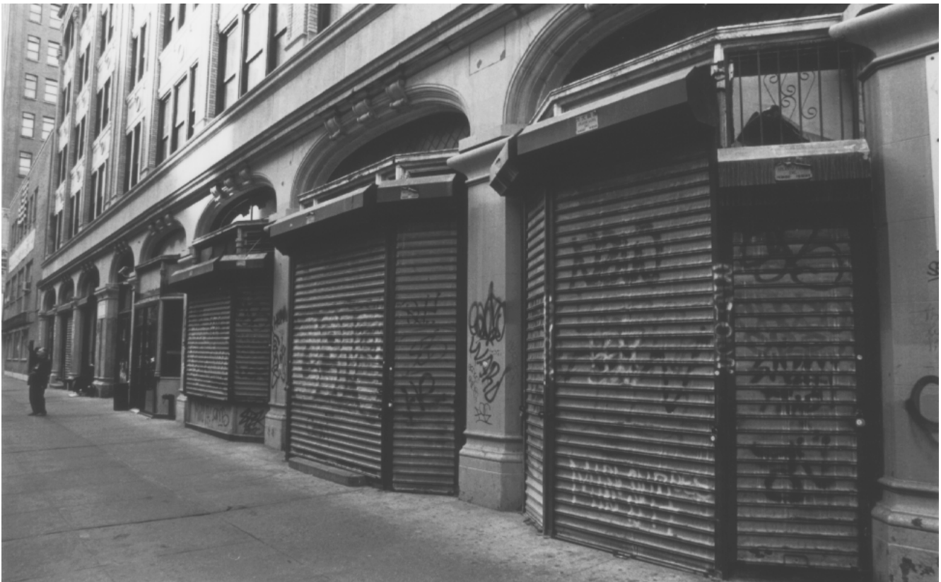
Detail of Lafayette Street Storefronts
